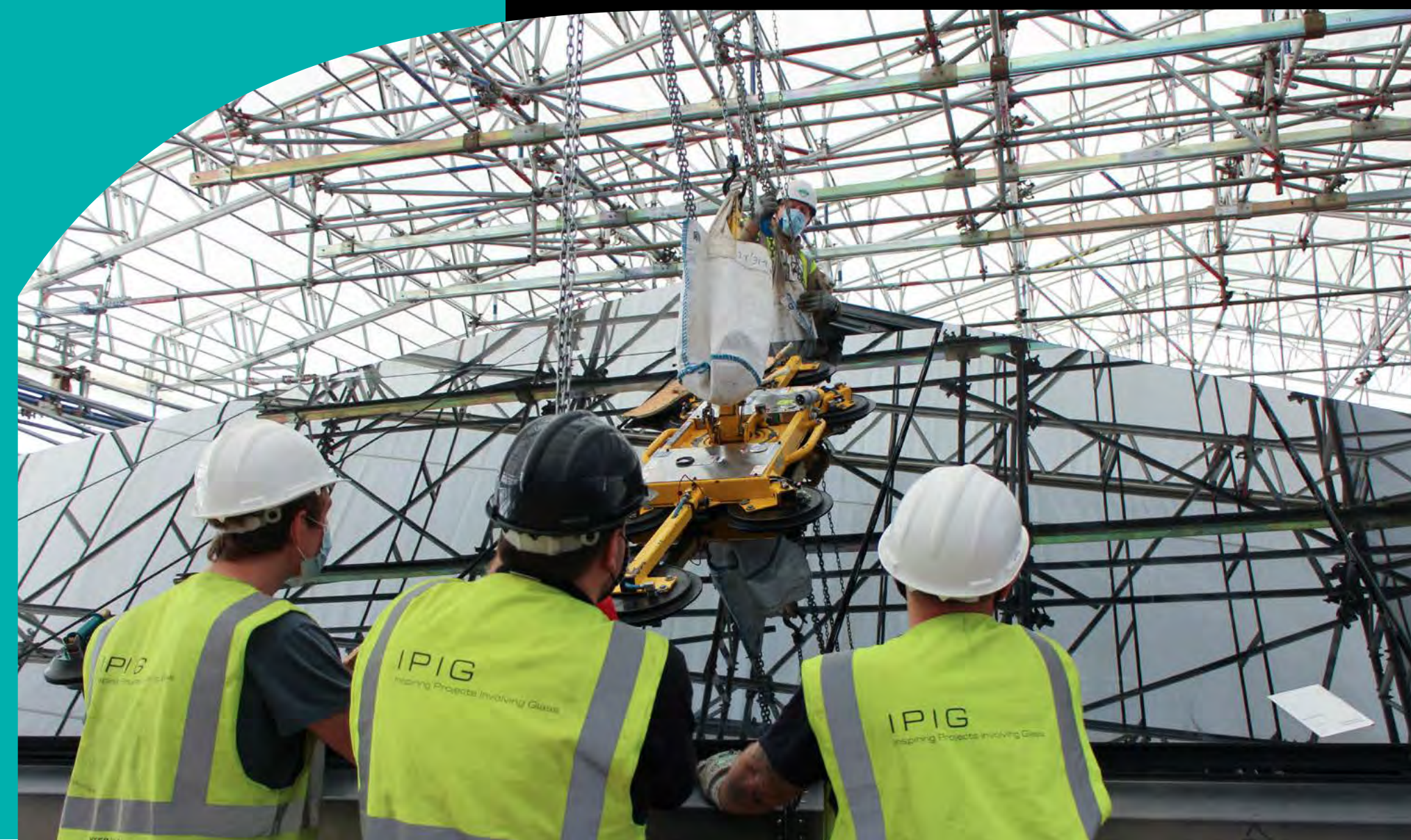
Top: Closed for redevelopment; Left: Installing the new skylight
